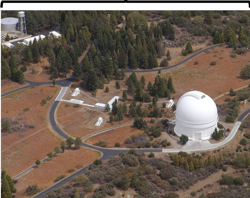
Palomar Testbed Interferometer, CA Three 40 cm apertures 110 m max baseline
